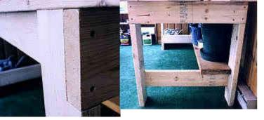
1 box of #7 screws 2 1/2". I used those black drywall screws because of their superior holding power.
